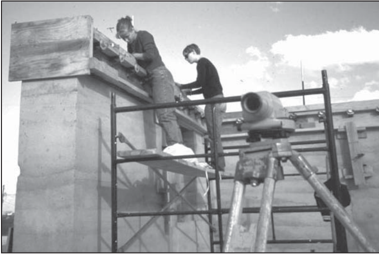
Figure 7. Bond-beam forms supported by pipe clamps put through wall at consistent height to ease the leveling process
