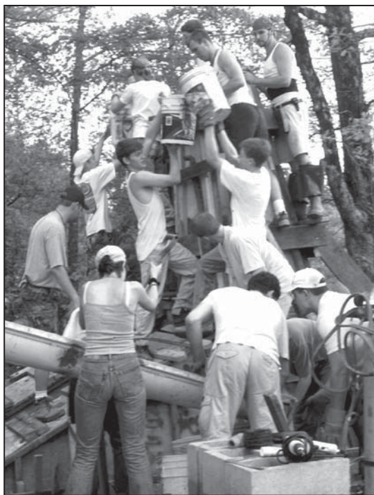
Figure 2. Pouring of concrete abutment for a pedestrian bridge in Chester, Arkansas
