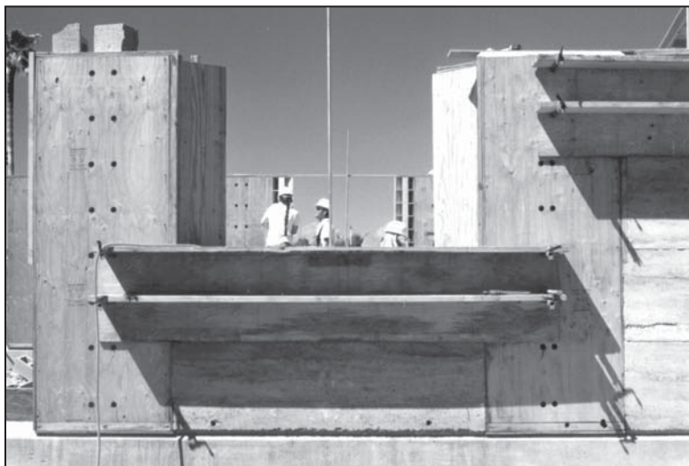
Figure 2. Incremental rammed earth forms assembled using simple elements
