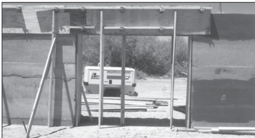
Figure 6. “Flying formwork” for bond beam was difficult to support and level.
