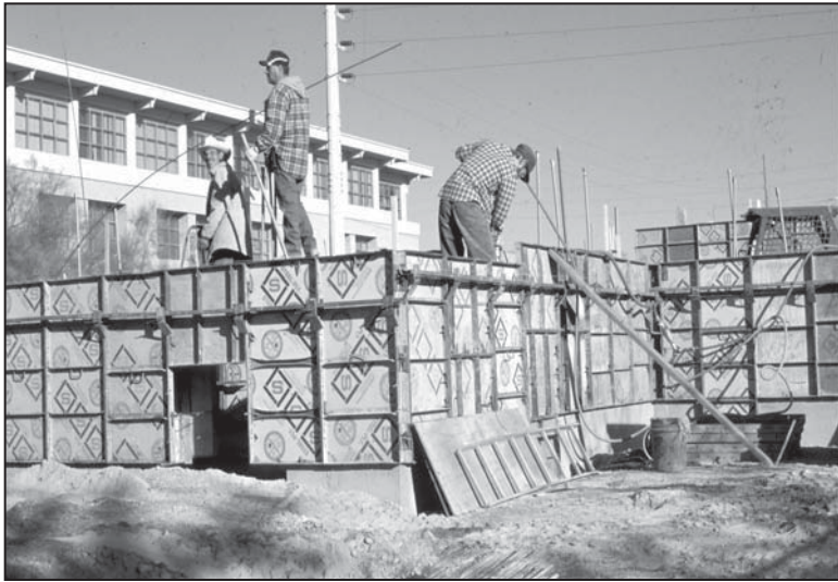
Figure 1. Conventional method of forming rammed earth walls using heavy, steel-reinforced forms.
