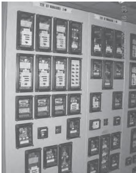
Fig. 4.1(a) Old distance relay scheme
