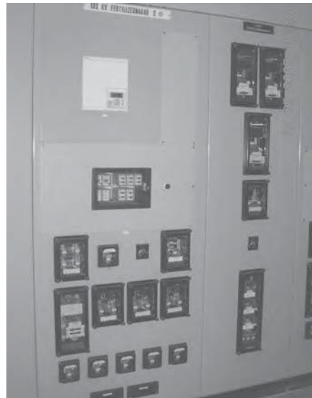
Fig. 4.1(b) Numerical distance relay scheme
