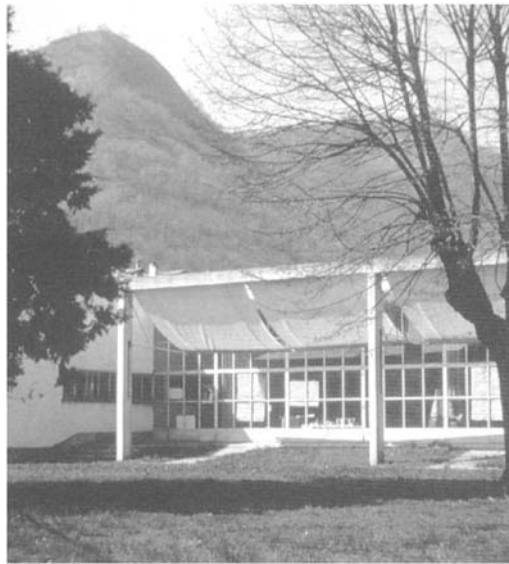
Figure 12.1 South-east façade with the classrooms and fabric canopies, following restoration
