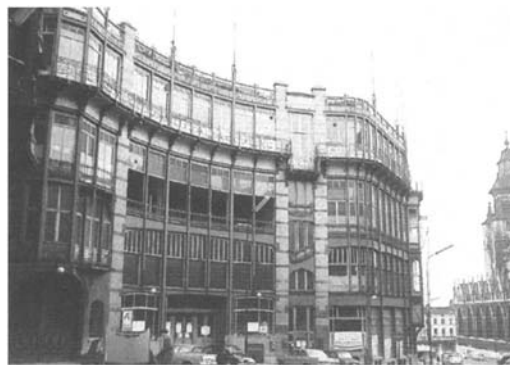
Figure 9.2 In Victor Horta's design for the auditorium at the top of the Maison du Peuple, the iron frame was enclosed only by glass or by very thin panels held in iron frames. Its Art Nouveau style strove for lightness, attenuation, and transparency; qualities that were easily expressed by metal and glass on the exterior
