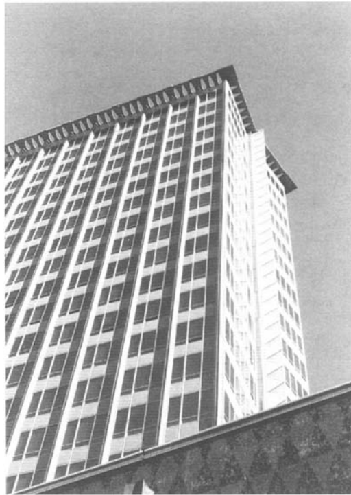
Figure 6.9 The BC Hydro Building (1955–57, Thompson Berwick and Pratt) has a unique lozenge shape with a reinforced concrete core located at the centre of the building that supports the cantilevered floors. A glass and metal spandrel curtain wall is also supported by thin metal piers on the exterior curtain wall. Mosaic tile murals are used at the base and in the interior lobby areas as public art. Listed on the Vancouver Heritage Register, this building was Vancouver's first designated Recent Landmark. It is a candidate for the DOCOMOMO International Register with the adjacent Dal Grauer Substation (see Figure 6.5 )
