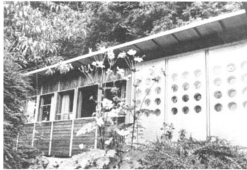
Figure 17.4 Perforated aluminium panels to service rooms and window panels to the bedrooms
