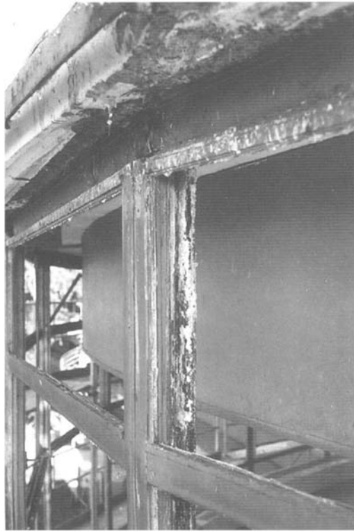
Figure 13.18 The appearance of the rotunda roof profile and window sections during restoration
