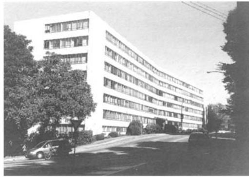
Figure 6.3 Hycroft Towers (Semmens and Simpson Architects, 1950) is a good example of the International style with a nonload-bearing screen wall made of alternating bands of metal spandrel panels and flush metal frame windows
