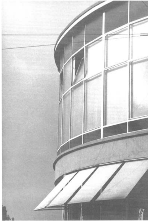
Figure 13.19 The rotunda façade after restoration—partial view. Restoring ironwork is a bit of a lottery. The rusty conditions of the standard sections, especially at the bottom of the glazing, condemned them from the outset. Given the real test where the thermal conditions of the building, especially in summer, do not impose additional constraints, it is possible to retain the existing sections provided the work is done on site to substitute the lower elements and then sandblast, protecting the profiles, before applying the final coat of paint
