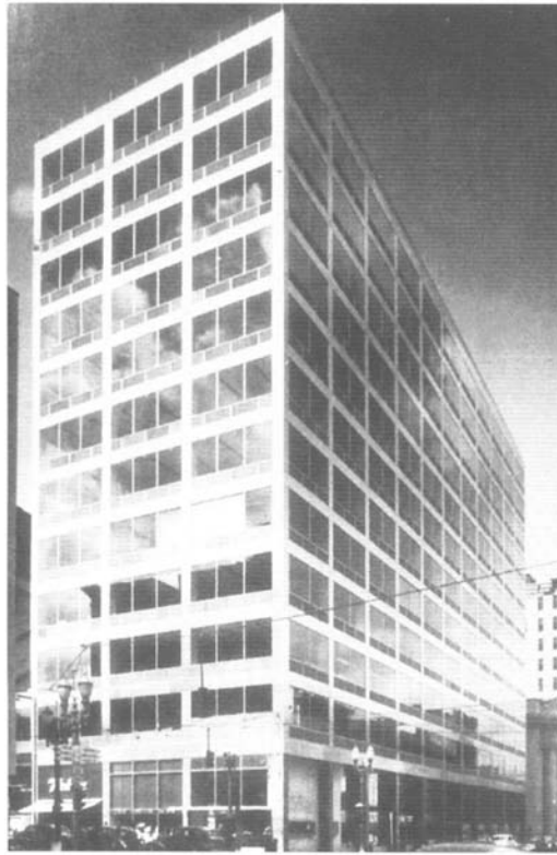
Figure 9.4 One of the first post-war buildings to be constructed with a glass envelope is the Equitable building (Pietro Belluschi, 1948) in Portland, Oregon. The Northwest US offered inexpensive power sources and airplane production facilities left over from World War Two. The Equitable Building was constructed with cladding panels made from rolled sheets of aluminum, and glazing frames which were simple extruded shapes. It was an early use of insulated glass
