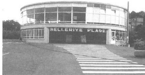
Figure 13.24 View of rotunda after restoration. Restoring the original roof profile and ensuring water tightness brought with it some surprises leading us to shed preconceptions. The roof had probably not been watertight for thirty years and the additional aluminium roof raised above the original by 50 centimetres on a wooden substructure allowed water to infiltrate around the edges of the roof slab. In addition, the false ceiling concealed and blocked the pipes ventilating the roofing surface. All these conditions combined to reduce the concrete around the edges of the slab to powder, requiring extensive reconstruction. In order to achieve a façade having due dignity it was simply a question of studying the very first photographs. It was necessary to free the façade of the neon, reconstruct the sign over the entrance and restore the curved security grille which, every morning in the summer, disappears into the ground as if by magic
