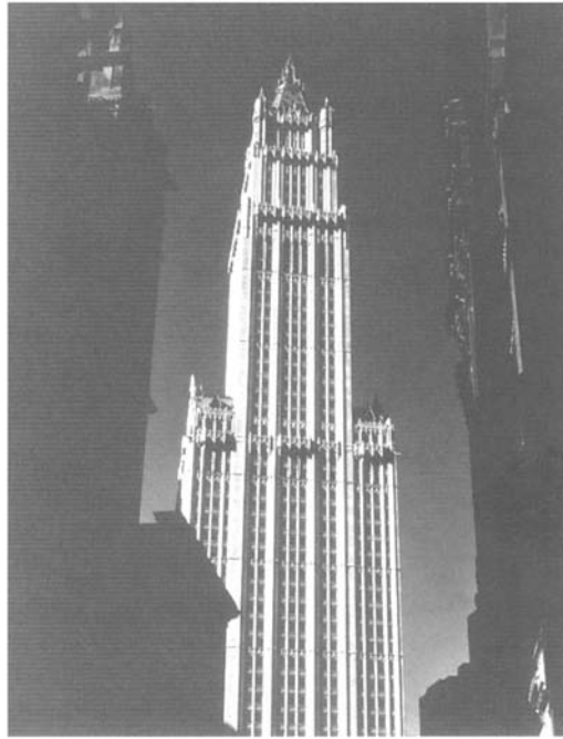
Figure 10.5 Woolworth Building, New York City. Architect: Cass Gilbert, 1913. Exterior view. Photograph by Theodore H.M. Prudon, 1981. While the contrast between old and new is rather evident from relatively close distance, further away the design intent of the original tourelles is fully met by the new tourelles. The overall appearance of the tower remains intact without the need for historic refabrication
