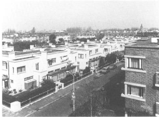
Figure 8.4 The Hague, Papaverhof, middle-class housing estate for the housing corporation ‘Duin en Daal’, designed in 1920–22 by the De Stijl architect Jan Wils with partial use of concrete walls; restored in 1989–90 with reconstruction of the original colour scheme
