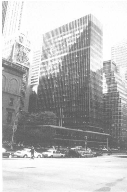
Figure 10.6 Lever House, Park Avenue, New York City. Architect: Gordon Bunshaft, Skidmore Owings and Merrill, 1952. Photograph by Theodore Prudon 1996. The successive failure of original spandrel glazing and related sections has resulted in a gradual replacement. The overall effect is a diminishing of the visual consistency of the design intent. The repair and replacement necessary and presently contemplated will ultimately result in an appearance that visualises the expectations of the original design intent but with only a very small portion of the original fabric remaining
