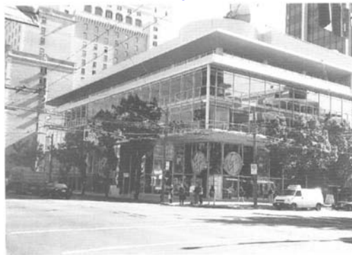
Figure 6.10 The rehabilitation of the former Vancouver Public Library shows the addition of a penthouse level, satellite dish and some of the neon signage. The sunscreen louvers on the Robson Street (right hand) facade have been removed. The curtain wall glazing has been sympathetically replaced with new double glazed panels in aluminum mullions which match the originals
