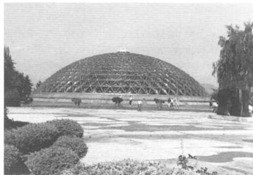
Figure 6.7 This triodetic dome is notable for its sculptural form and roof structure. The roof on the Bloedel Conservatory (Underwood McKinley Cameron Wilson Smith and Associates, 1969) consists of triangular frame elements of aluminum pipe infilled by plexiglass panels. Listed on the Vancouver Heritage Register
