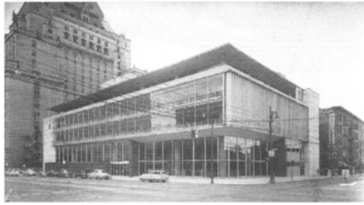
Figure 6.1 The Vancouver Public Library (Semmens and Simpson Architects, 1956–57, is a very good example of an institutional building from the Modern Period. Some of the building's more notable design features include a reinforced concrete structural system with curtain wall glazing creating an open interior design, a distinctive perimeter cantilever and roof projection with a knife edge profile and a unique two-storey glazed corner at street level that provides openness and encourages public accessibility. The Vancouver Public Library was also one of the first in the city to incorporate public art in the design of the building. The building was rehabilitated for retail, restaurant and TV studio uses in 1995–97. See Figure 6.10 . Listed on the Vancouver Heritage Register and a municipally designated building. Archival photo c. 1958 courtesy Vancouver Public Library
