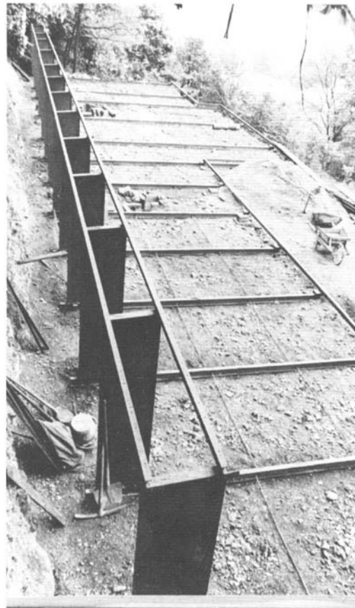
Figure 17.2 North façade double frames of metal profiles on the retained, excavated platform
