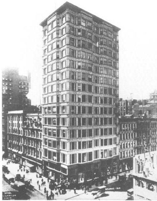
Figure 9.1 An archetype of the Chicago School and example of the structural innovations of the late nineteenth century can be found in the Reliance Building. The Reliance Building curtain wall of terracotta, a masonry material, is a clear aesthetic expression of the underlying structure and provides a maximum of natural lighting. This facade treatment has been compared to the 1921 'Glass Skyscraper,' study project of Ludwig Mies van der Rohe
