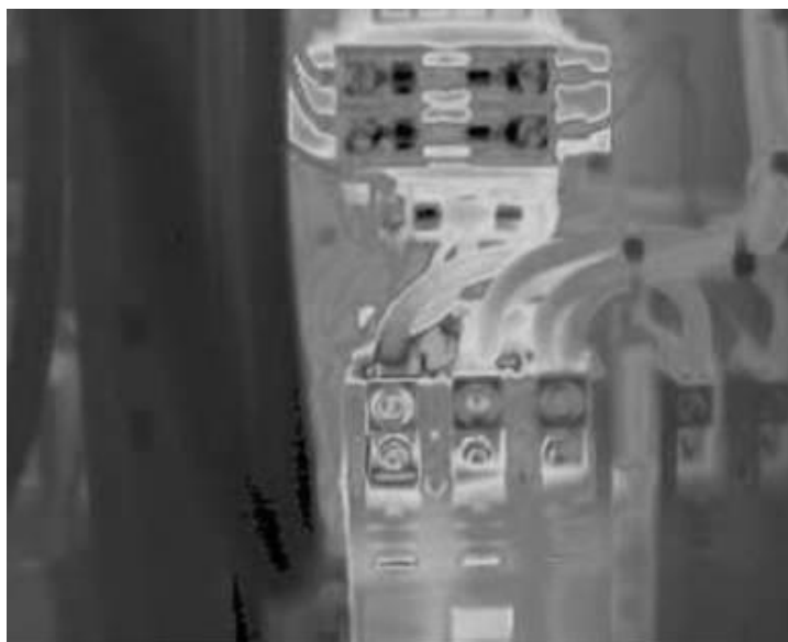
Figure 7.2-6. Loose Connection on A-Phase in a 2 Speed Motor Contactor
