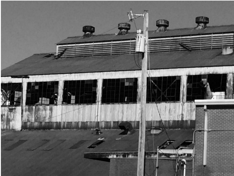
Figure 7.1-4. Chemical Plant Shelter Showing Signs of Severe Deterioration
