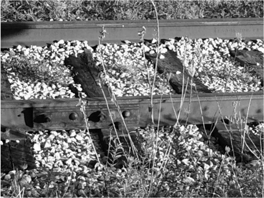
Figure 2.3-3. Rotted Railway Ties Providing Weakened Support
