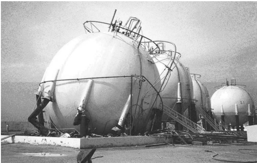
Figure 7.1-3. Liquefied Petroleum Gas (LPG) Storage Sphere Collapsed While Being Filled for a Hydrostatic Pressure Test
