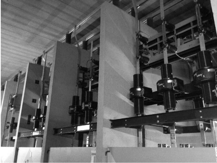
Figure 7.2-7. Medium Voltage (15kV) Indoor Open-Air Switchgear
