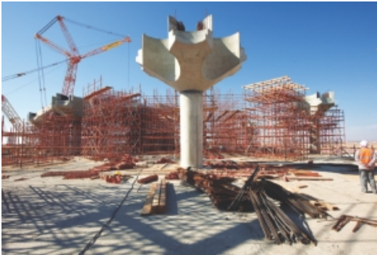
Figure 15.9 Queen Alia Airport, prefabricated concrete column heads installed on site. (Image credit Nigel Young/Foster + Partners, copyright Foster + Partners.)
