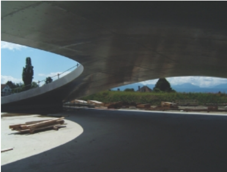
Figure 17.2 EPFL Roles Learning Centre concrete shell. (Reproduced by permission of Bollinger + Grohmann.)
