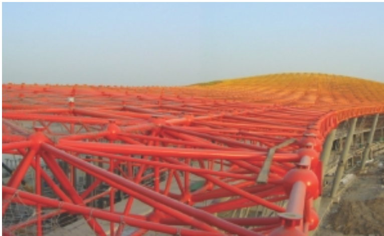
Figure 15.4 Beijing Airport, spraceframe structure under construction. (Image credit and copyright Foster + Partners.)
