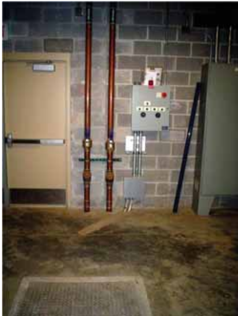
Figure 7-4 Coverdell Building storage cistern (access hatch and piping).
