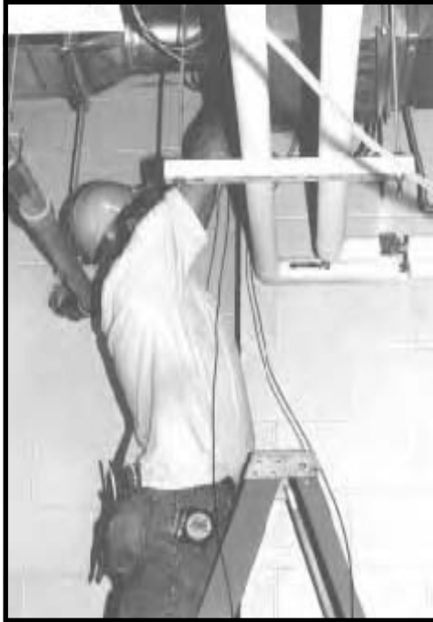
Figure 22-4. Construction worker using fiberglass ladder around electrical conductors.
