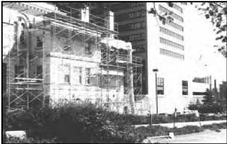
Figure 22-3. During this type of construction activity, falls, struck-by, moving objects, tripping, structural collapse, or material handling incidents could occur.
