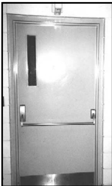
Figure 16-4. Common or typical exit door with a panic bar.
