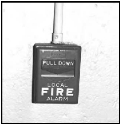
Figure 17-5. A pull-down to activate the fire alarm.
