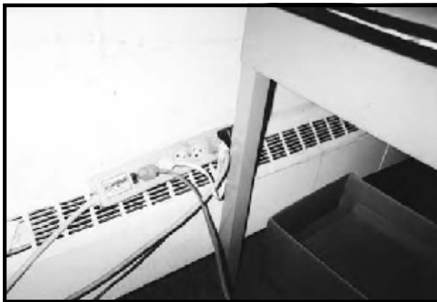
Figure 7-2. Electric cords wedged against a heating unit.
