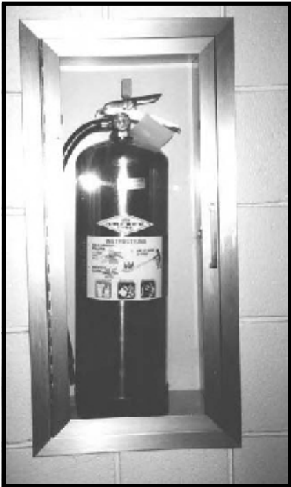
Figure 17-2. Make sure that all fire extinguishers are in working order and have been inspected monthly.
