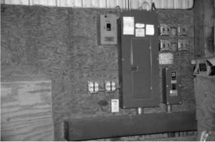
Figure 16.28. Electric service will require a subpanel to accommodate the electrical load requirements of indoor arena electric lights. The subpanel area should be inaccessible to horses at all times including for loose horses in the arena. Use covered convenience outlet and switch fixtures (not shown here).
