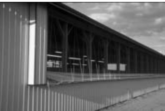
Figure 6.19. Strong, translucent curtain material is raised and lowered over the top portion of the sidewall. Permanently open eave vents on top of curtain provide ventilation even when curtains are fully closed during colder weather.
