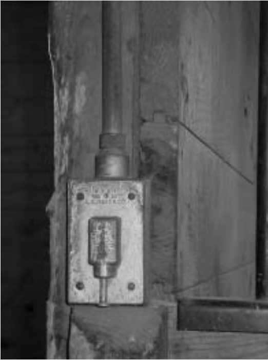
Figure 10.1. Example of a rugged, horse-proof switch located just outside stall in area accessible by the horse, as evidenced by chewing marks on wood support. Light switch is a stem that moves in and out of fixture from lower edge. Use this type or similar fixture to protect horse from electrical shock and prevent horse actuation of lights.
