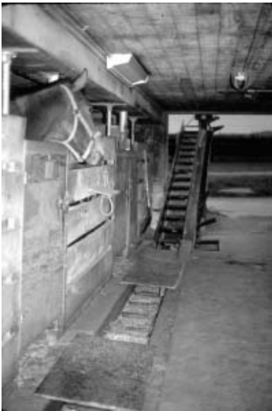
Figure 8.9. Some converted traditional dairy barns will have an operating manure gutter cleaner that can be converted for horse stall waste transport.
