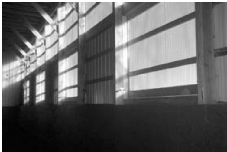
Figure 11.5. Translucent panels used in indoor riding arena for light entry. This arena has two sides surrounded by stabling that results in a limited area for natural light entry compared with a free-standing arena. A good solution was the addition of the extra translucent panels along one sidewall. These panels slide open for fresh air entry.
