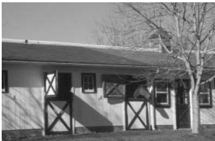
Figure 6.1. Horse stables have obvious door and window openings to maintain fresh-air conditions during most weather. This stable also provides openings that are always open at the ridge vent and cupola and along the eaves of the building so that even during the coldest weather, when doors and windows are closed, there is still some fresh air exchange.
