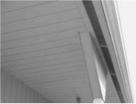
Figure 6.12. Eave vents protected with wire mesh of large openings are a good option to provide for fresh air into stables during all weather. Here the 4-inch opening on the breezeway soffit is matched by an equal-sized opening on the opposite sidewall eave.
