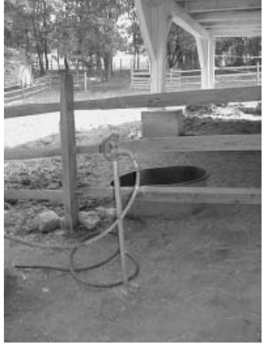
Figure 10.12. Outdoor horse watering tank with nearby frost-proof hydrant for convenient filling year round.
