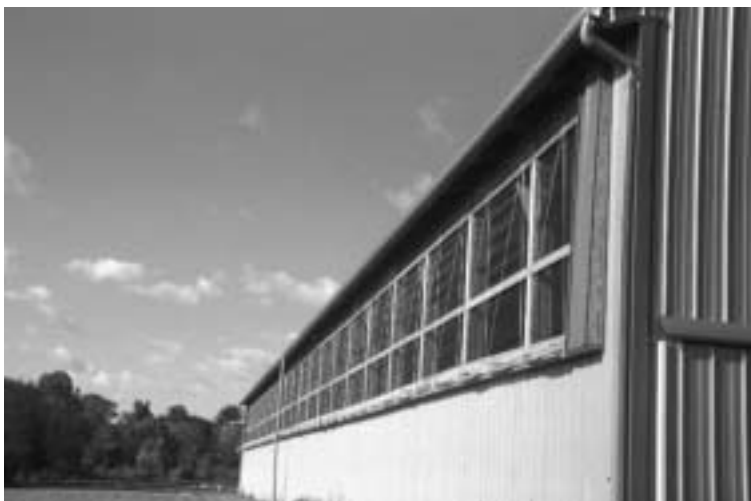
Figure 16.16. Curtain material as the upper portion of the sidewall can be used to easily provide large fresh air and light openings. They typically open from the top down.
