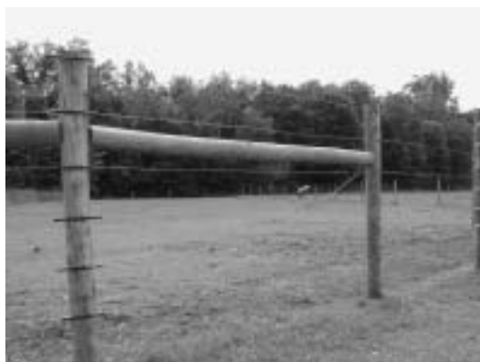
Figure 15.11. High-tensile wire fence offers the advantage of wider post spacing than conventional wire fence, shown here. Without electrification, several wire strands will be needed to contain horses, such as the six-strand fence shown here.
