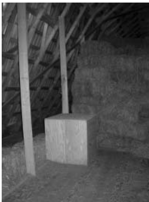
Figure 13.6. Plywood box covers hay drop hole for greater safety than leaving an open hole. Hay can be stacked around and over the box, which is open facing the roof wall.
