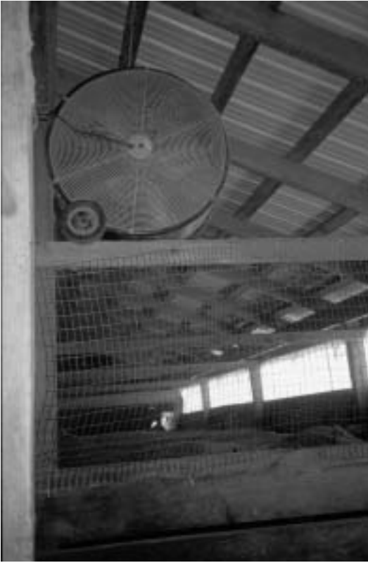
Figure 6.8. Stables without adequate air movement can use circulation fans to supply wind speed over horses in key locations. Choose fans that have motors and components that can tolerate the dust and humidity of horse stables. Fans, such as the one shown, are marketed to the agricultural and horticultural markets.
