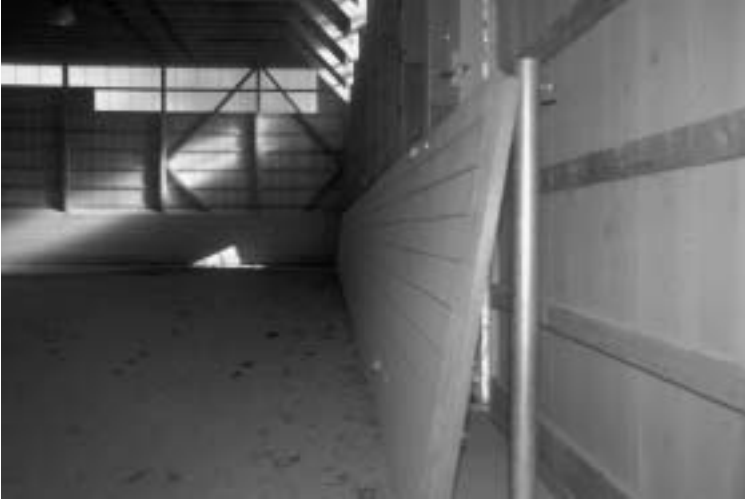
Figure 16.25. Movable arena rider guard protects riders at large sidewall door opening. Post supports both halves of the swinging guard when closed.
