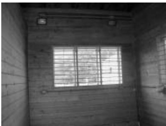
Figure 10.6. Overhead lights in wash stall and veterinary care area are located at back of stall and in similar position at front opening. Electrical wiring is protected in PVC conduit with moisture-proof fixtures on lights, junction box, and convenience outlet. Note protective bars on windows, which admit plenty of natural light, and rugged wood wall construction.
