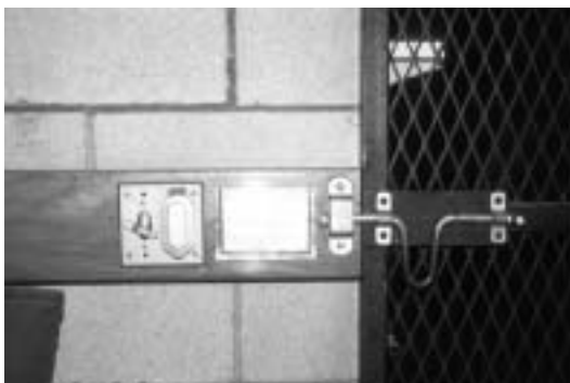
Figure 5.9. Strong secure hardware and protected electrical components are needed around horse stables. Many facilities provide information about horse identity and care conveniently located near each stall door.
