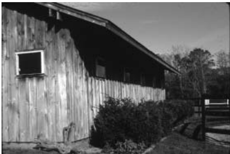
Figure 11.4. Stable windows shaded from excessive sunlight entry and glare during warm weather.
