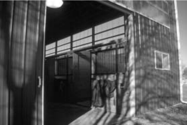
Figure 11.1. Light entry in a stable combines natural light, shown here via windows and translucent siding panels, and electric light, via HID light fixtures in this photo.
