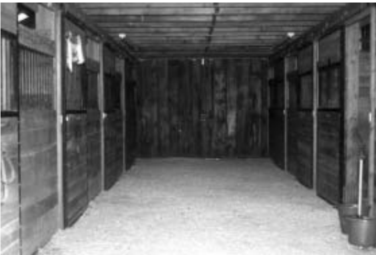
Figure 2.5. Center aisle design, with its enclosed, weather-protected work aisle with stalls on either side, is very common in the United States. This stable features hay storage over the center aisle with no ceiling over the horse stalls.
