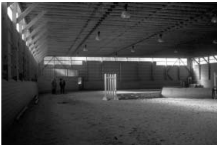
Figure 16.21. Natural lighting via translucent panels located on all four sides of the indoor arena. An elevated platform in a corner offers a relatively inexpensive construction that allows spectators a good view of arena activity. Storage is provided under the platform for training aids, and so forth.
