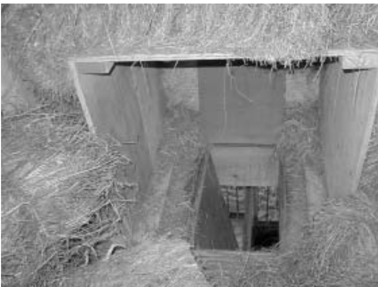
Figure 13.8. Interior of same plywood box shown in Figure 13.7 but with hinged baffle in second position to divert hay delivery to stall on the right.
