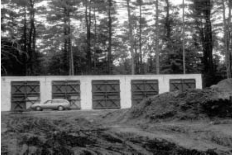
Figure 8.22. Composting facility where bunker rooms contain horse stall waste subjected to forced aeration to speed process versus static pile composting. Finished compost is stockpiled in the foreground.
