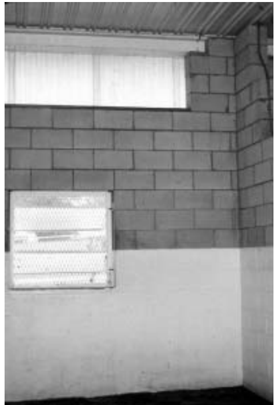
Figure 3.13. Sealant is used on lower portions of masonry stall wall construction to assist in cleaning.
