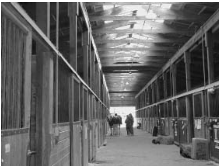
Figure 11.6. Although not generally recommended because of challenges of maintaining a leak-free construction and uncontrollable solar heat gain, roof translucent panels offer a naturally bright interior to this four-stall-wide fairground stable.
