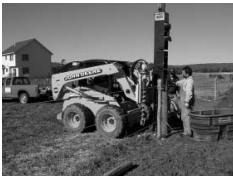
Figure 15.22. Driven posts offer stability from compacted soil around the post as it is driven into the ground. Photo courtesy of Jennifer Zajackowski.
