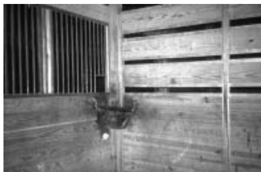
Figure 5.14. Gaps for enhanced airflow formed by spaced boards on stall wall. Boards protected from chewing with metal edges.
