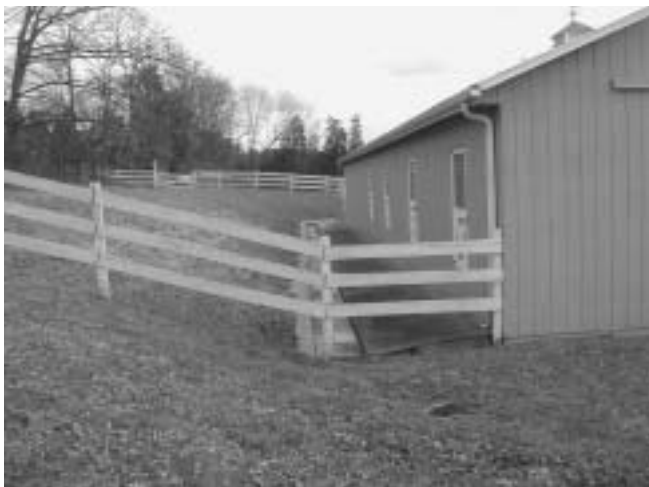
Figure 4.4. This stable was best positioned into a small slope because of drainage challenges at other more level, but lower, sites on the property. A shallow trench lined with concrete diverts surface water and downspout water away from the building foundation and discharges it on the downhill side of the structure via underground pipes.
