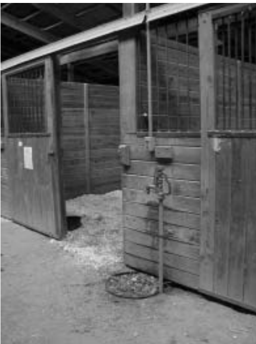
Figure 10.7. Frost-proof, self-draining water hydrant in unheated stable secured to nearby wall with overflow drainage area.
