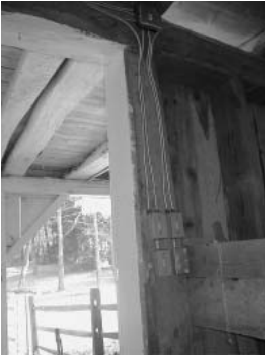
Figure 10.3. Electrical service in older barns converted to horse stabling, such as this classic bank barn formerly housing dairy cattle, need to include safe wiring. Here metal conduit and moisture-proof switches and outlets are located away from horse contact.
