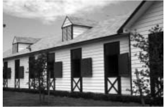
Figure 6.29. This stable offers ridge ventilation via louvered horizontal "cupolas" on the roof design. Mild weather fresh air is admitted to each stall via Dutch doors with top portion open, as shown. When the bottom portion is likewise opened, a full-screen mesh door prevents the horse from exiting while allowing entry of plenty of fresh air. Glass plastic panels above each door admit light year round.
