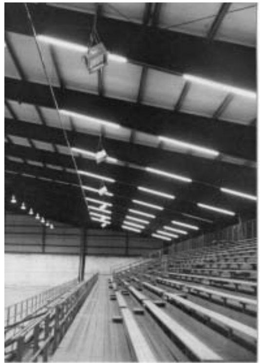
Figure 16.19. Radiant heaters are used to heat occupants of the arena at key locations, such as a spectator area. Courtesy of Detroit Radiant.
