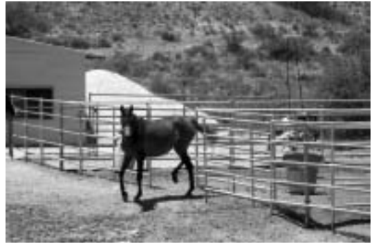
Figure 15.18. Metal pipe and cable fences are sturdy and affordable alternatives to wood board fence in areas of limited lumber supply.
