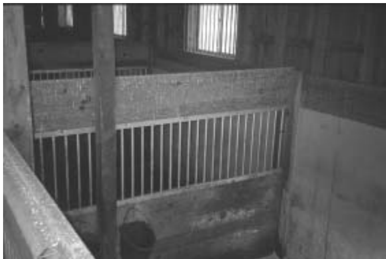
Figure 3.11. Poured concrete exterior wall of this stable is mainly below grade on this bank-barn construction.
