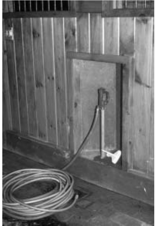
Figure 10.8. Self-draining water hydrant recessed into stable aisle wall for additional safety from horse impact.
