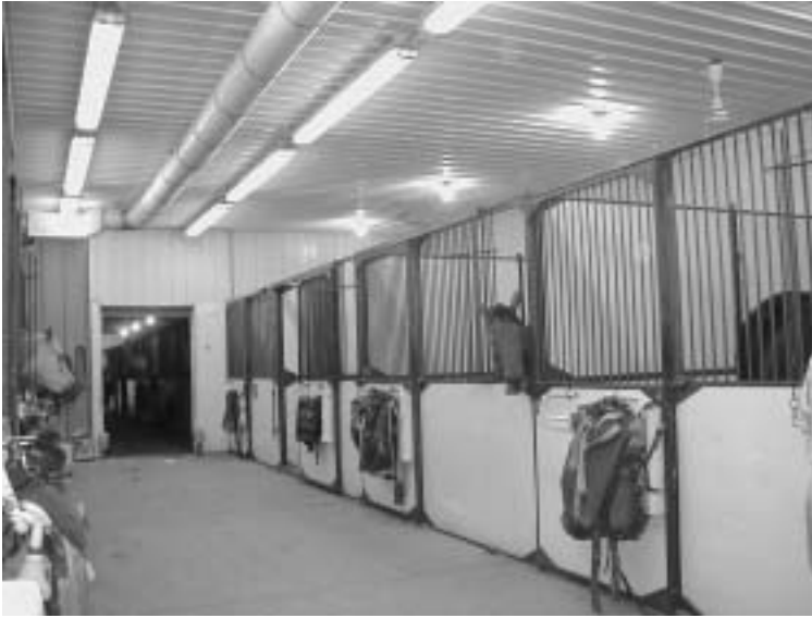
Figure 12.8. Heated stable with overhead rigid duct that delivers warmed air throughout the stable interior. The heater is located nearby in a separate utility room.
