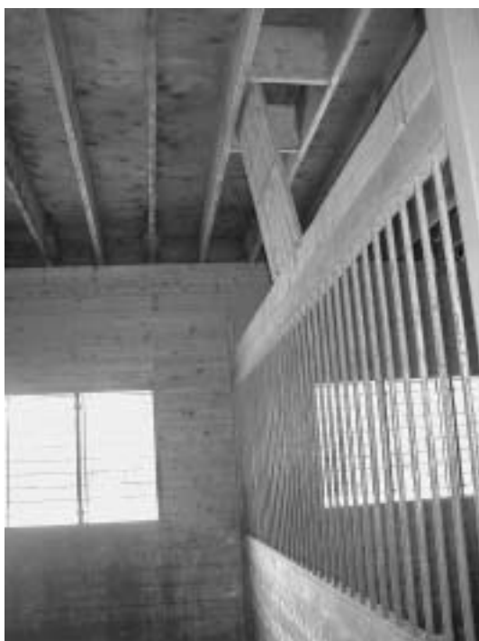
Figure 13.9. View of haymow drop design where baffle board is seen to be hinged from the top of the stall divider.
