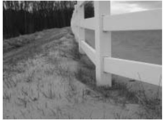
Figure 18.9. Outdoor arena surface will need frequent conditioning to keep the loose footing material evenly redistributed from the effects of horse traffic and water runoff that throw or flow, respectively, the material just outside the arena perimeter.
