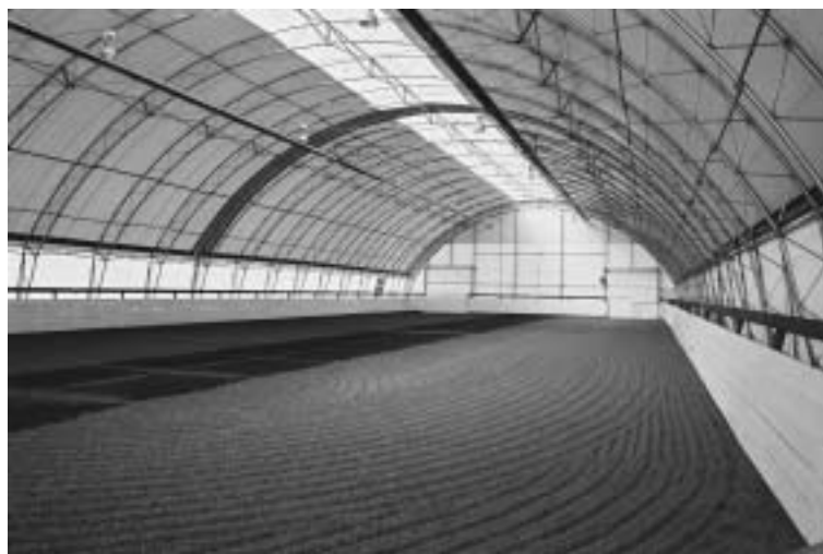
Figure 16.10. Hoop structures covered with a flexible material offer clear-span construction. Courtesy of Coverall Building Systems.
