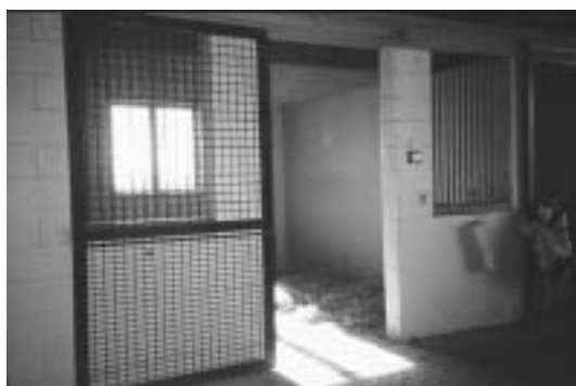
Figure 5.8. Concrete block stall wall construction with full screen sliding door.
