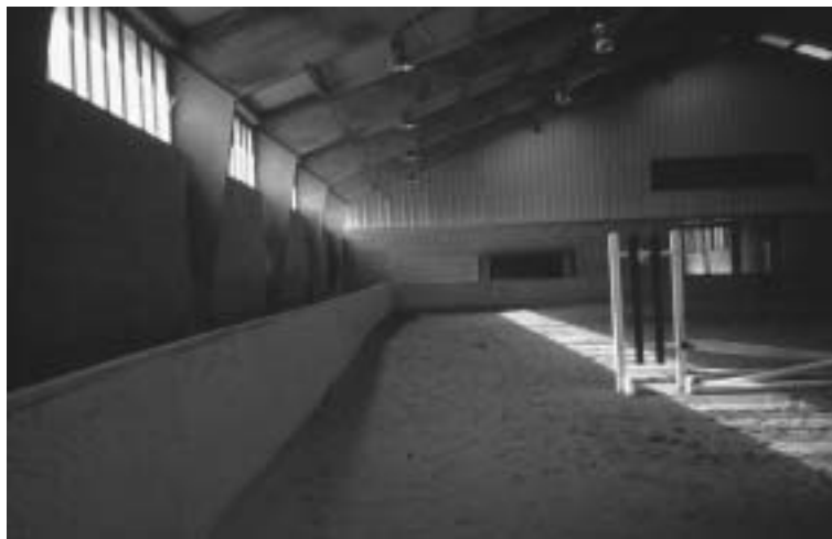
Figure 16.9. Rigid-frame clear-span construction is common in larger indoor arenas.
