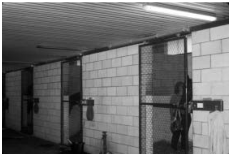
Figure 6.35. For stable designs that chose to have solid sidewalls, and in this case solid front walls, the ability to get fresh air into each stall is limited. In these cases use full mesh doors, high ceilings, windows, and eave and ridge joints to ensure fresh air entry to each stall to provide as much internal air distribution as possible.
