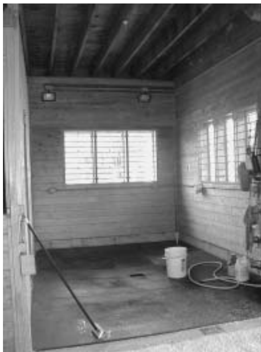
Figure 13.19. Rubber floor mat as floor of wash stall that has stained wood lining, natural light from windows protected by bars, and sealed light fixtures in front (not in view) and rear of wash stall.
