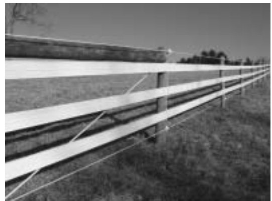
Figure 15.19. A flexible vinyl rail installation that mimics the appearance of board fencing is proving to be a safe and low-maintenance alternative with some installation savings with wider post spacing.
