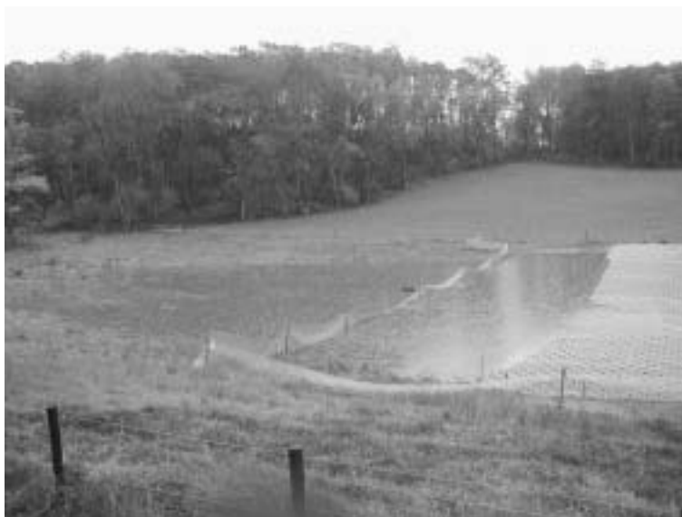
Figure 4.7. Paver blocks interlace for a strong, permeable surface (shown here) recently installed in a groundwater recharge basin in a horse pasture. The temporary fence was removed before horses were allowed back into the pasture. Courtesy of Larry Fennessey.
