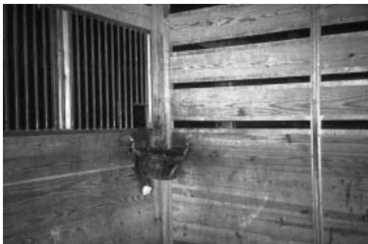
Figure 6.34. Stall wall with gaps for improved air movement within the stable when solid walls are used between stalls.
