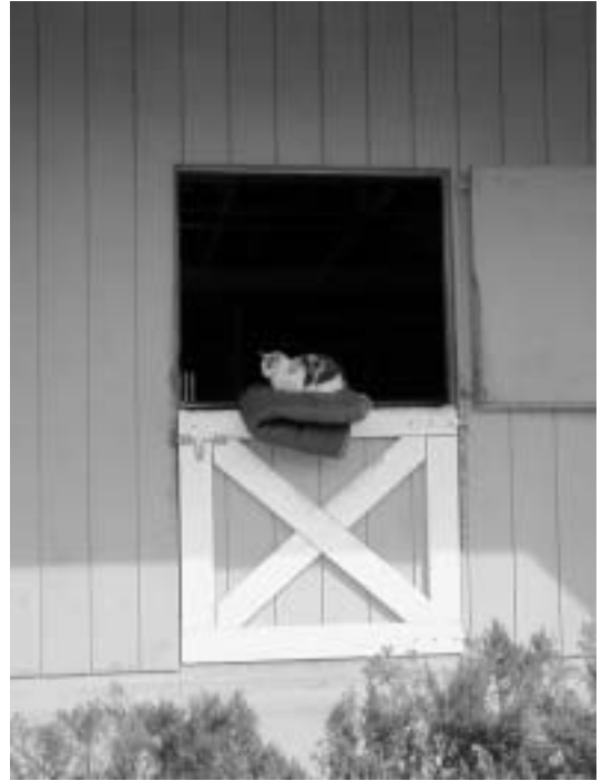
Figure 5.6. Dutch doors are popular horse stable door construction because horses are able to look or reach outside while contained by the lower door partition.
