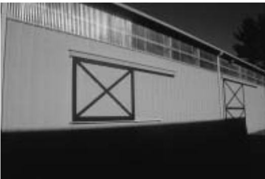
Figure 16.15. Sliding doors and panels are popular for providing large openings for admitting summer breezes to the arena.
