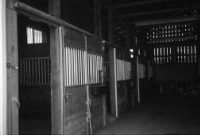
Figure 6.32. Stable interior showing airflow gaps of the breathable wall siding at end of stable aisle. This stable has other good ventilation features, including eave and ridge vents, a window that opens for each stall, open grillwork on stall partitions, and no overhead airflow obstructions.
