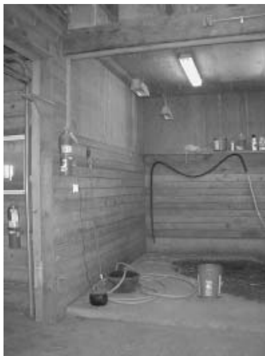
Figure 13.18. Wood kick board liner on lower portion of wall of combination grooming station/wash stall area. Note hanging radiant heaters and sealed fluorescent light fixture.
