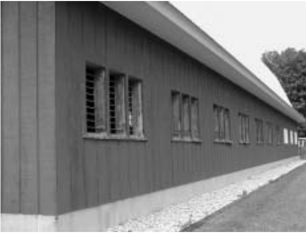
Figure 4.6. Rain run-off and snowmelt from large roofed areas can be handled without gutters and downspouts in cold climates with provision for capturing and diverting large amounts of water at the foundation base, as shown here with a wide swath of graveled French drain.
