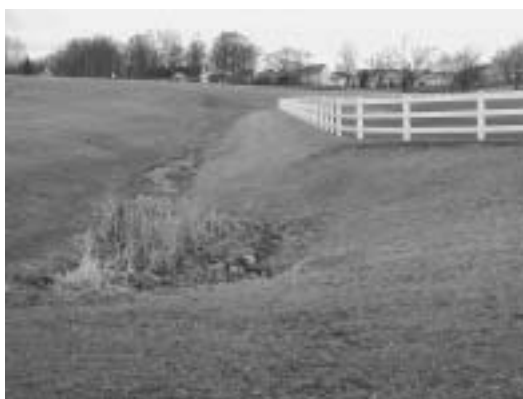
Figure 18.4. Divert surface water from the outdoor arena site with a swale or other suitable diversion.
