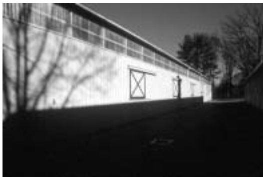
Figure 3.16. Translucent panels are popular as the upper portion of sidewall construction for admitting natural light to stables and indoor riding arenas.
