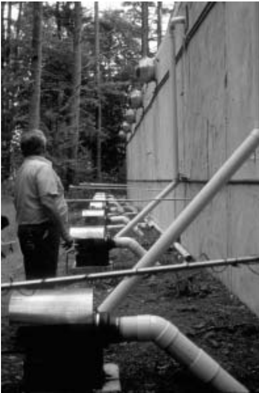
Figure 8.23. Fan, temperature instrumentation, and air distribution piping behind aerated bunker composting facility.
