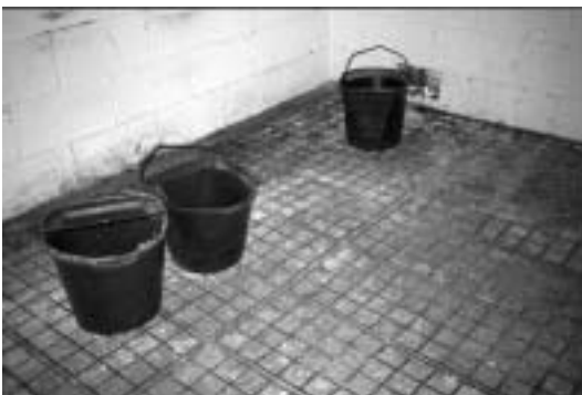
Figure 7.5. Clay material fills the space within the grid used in this floor at a veterinary facility.
