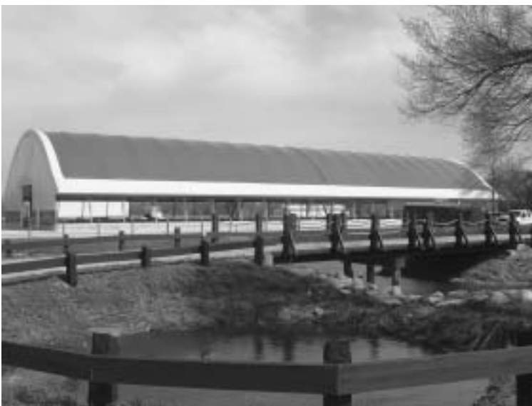
Figure 16.23. The translucent cover material of hoop structures is attractive for the abundant natural light interior. Select material that reduces glare and solar gain. Courtesy of Coverall Building Systems.
