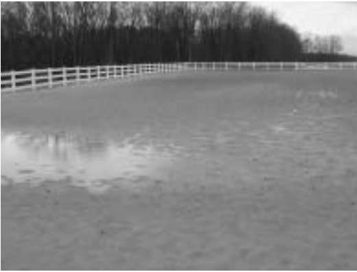
Figure 18.1. With inadequate crown (or slope) to the outdoor riding arena surface, water will pond in a low spot. Without adequate base preparation, low-lying areas form in locations of heavy arena use.
