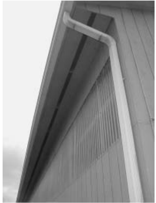
Figure 16.13. Provide eave openings along entire arena sidewall length. Protect opening from bird entry with nothing more restrictive to airflow than 1-inch square hardware wire mesh.
