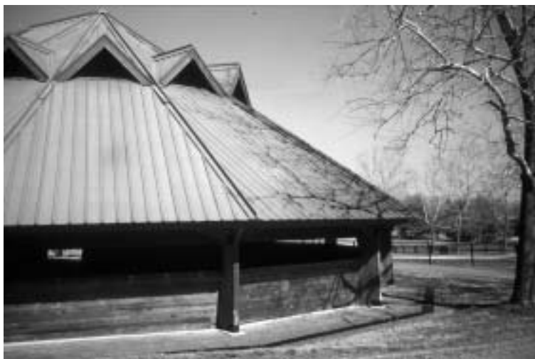
Figure 16.30. Drainage of a substantial amount of water from the arena roof is necessary. Where flat topography does not allow adequate gravity flow to a suitable location, an in-ground drainage system will be necessary.
