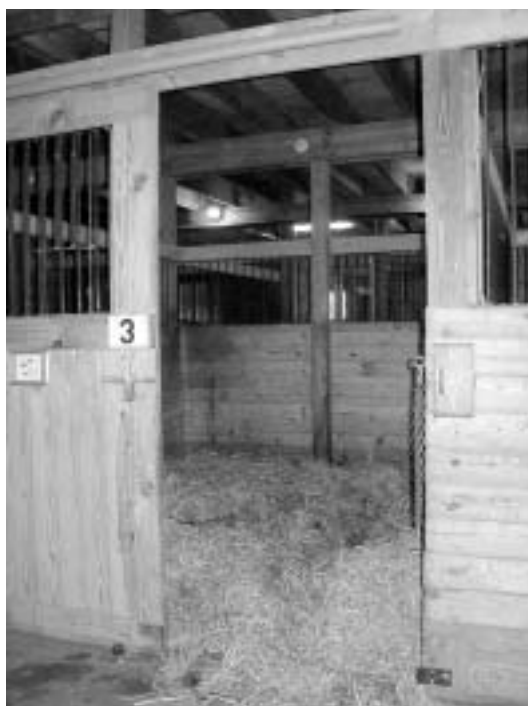
Figure 5.13. Rugged construction for horse stall is needed in material for walls and hardware for securing door. Pressure-treated bottom boards of wall are in contact with ground and manure. Open partition design allows enhanced visibility and ventilation air movement in this stable with two central aisles and four stalls across its width. Note smoke detector above back wall of stall.
