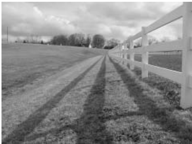
Figure 4.5. A vegetated diversion trench intercepts surface water from flooding an outdoor arena footing and saturating the base.
