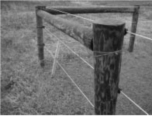
Figure 15.17. Polybraided wire and polytapes provide a visible, safe horse fence at lower cost than more traditional board and mesh fence installations. Photo courtesy of Jennifer Zajackowski and R&R Fencing.
