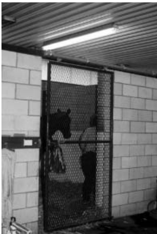
Figure 3.14. Concrete block masonry construction is more common as an exterior wall material but can also be used as stall partition.
