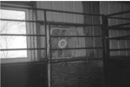
Figure 9.5. A fan designed for residential use, such as the “box” fan shown, has potential for motor to overheat because it does not have a fully enclosed motor and is not designed to remain cool under high dust accumulation. Agricultural grade fans are recommended for use in horse stables whether they are used for circulating air over individual horses in a stall or for exhaust of stale air.
