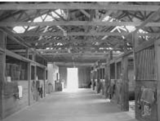
Figure 3.2. Clear-span construction uses trusses that provide an open interior. Stall corner posts attach to the lower chord of some trusses but are not supporting the roof weight.
