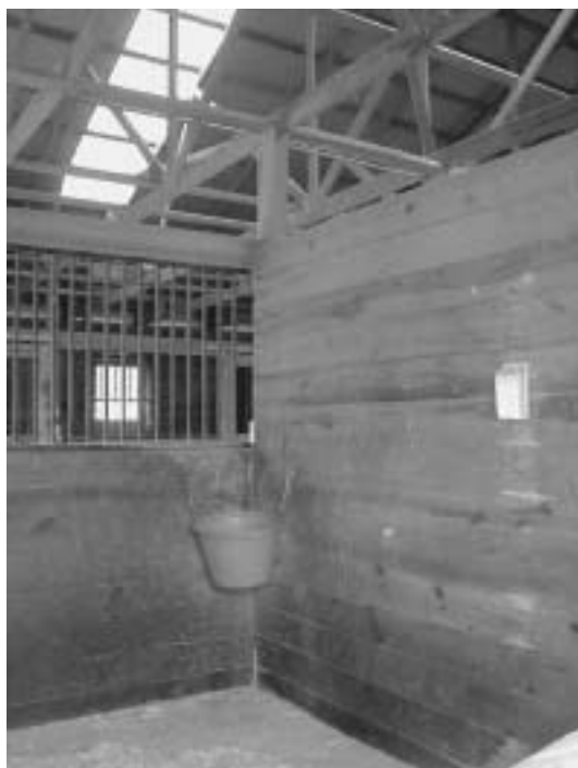
Figure 3.10. Wood is the most common material for stall wall construction. Wood is often used as a liner on the interior of masonry walls and is needed as a stall liner for metal-sided buildings.
