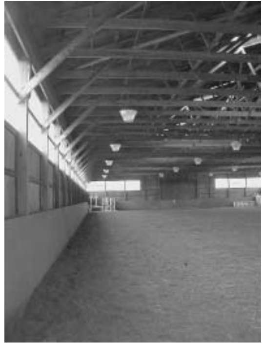
Figure 16.8. Trusses are used for clear-span construction in small- to medium-sized indoor arenas.
