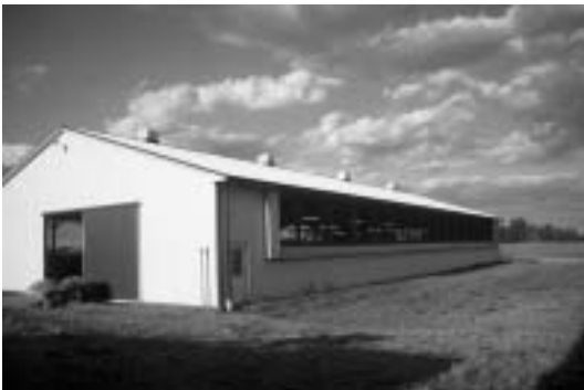
Figure 6.18. Stable with island design of stalls with exercise aisle around perimeter. Stable has sidewall curtains for air and light entry.
