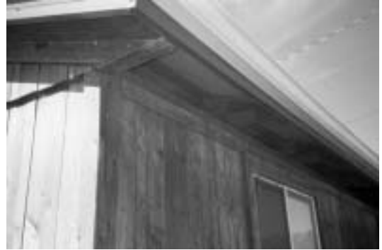
Figure 6.14. Do not be afraid to provide plenty of permanently open fresh air vents to the stable. This eave inlet is 13 inches wide, on a 16-inch overhang, on a 32-foot-wide stable in a cold climate. Ridge opening is also provided and the stable environment has excellent fresh air quality year round.
