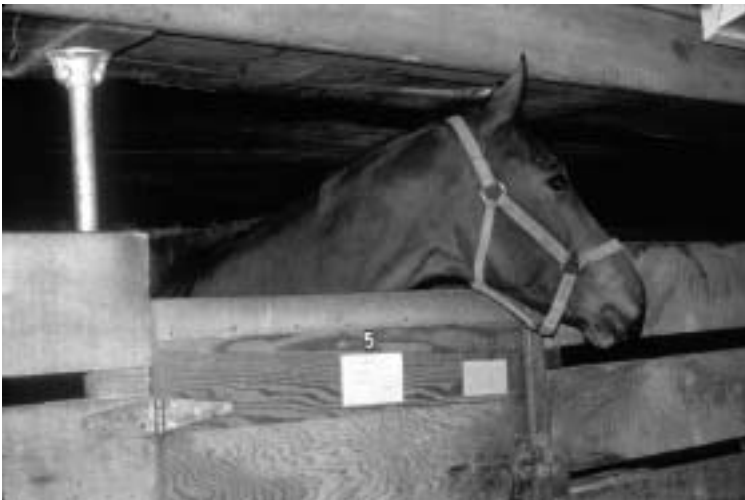
Figure 6.37. A low ceiling, as shown, is never deliberately designed into a horse stable; but with some old barn conversions, one is handicapped by original construction. Be sure to provide plenty of airflow via gaps between stall wall boards and ducted fresh air if necessary. In this case, the horses were not confined to the barn for long periods.
