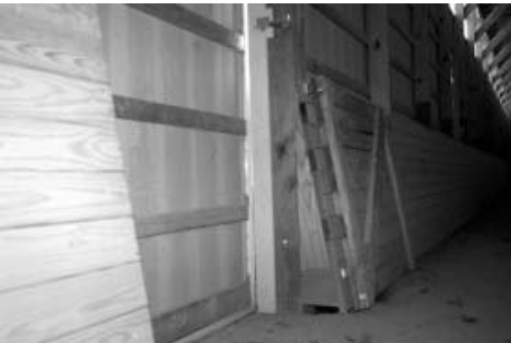
Figure 16.26. Rider guard is continuous around entire arena perimeter, so provision is made to have gated guard construction (shown here hinged back against the stationary guard) for accessing arena entry doors.
