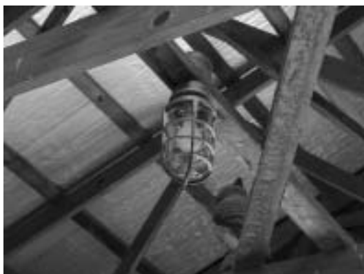
Figure 12.17. Roof insulation is useful even in unheated stables to decrease condensation by maintaining the interior surface temperature near interior air temperature. Insulation with reflective surface is shown, which can provide insulation value if kept shiny and facing an airspace.
