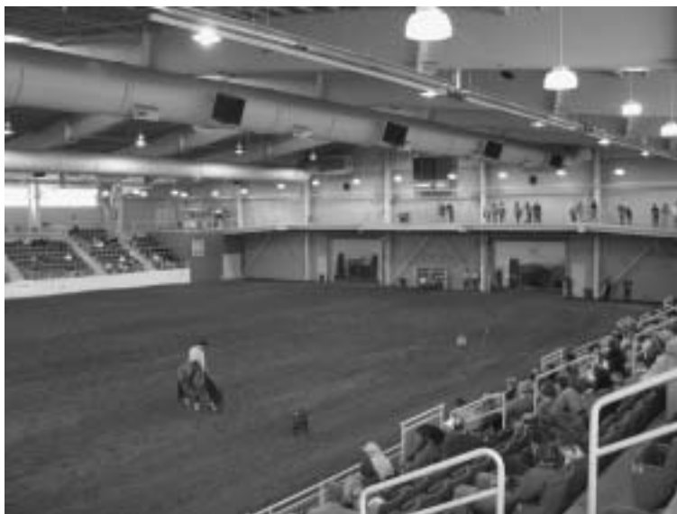
Figure 12.15. Long radiant tubes are positioned (near the overhead lights) to deliver heat to spectator area in addition to space heat supplied by the furnace ducts.
