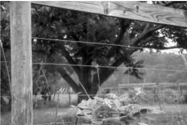
Figure 15.10. Wire strand fences suffer from poor visibility to the horse, so adding a top board or a thicker and bright material will improve safety. A top board offers the advantage of discouraging reach over the fence but limits the post spacing distance.
