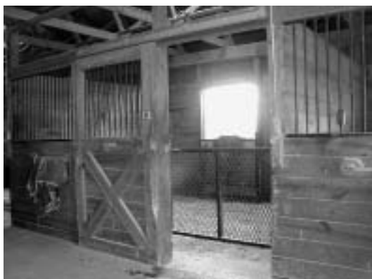
Figure 5.12. Stall with both interior and exterior doors, both of which have two doors. The primary exterior door is a Dutch door and the primary interior door is a sliding wooden door with bars on top portion. A half-screen door is provided at each location for increased airflow. Eave inlet allows fresh air exchange at back wall of stall.
