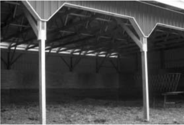
Figure 6.7. Sidewall openings on both sides of a building are key for natural ventilation function. Even an open-front shelter, with the whole front area opened, needs a back eave opening to ventilate properly.
