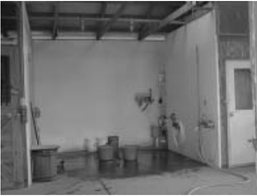
Figure 10.14. Horse wash stall water needs include hot and cold water supply and drain system for washwater and potentially a limited amount of manure waste. Area often doubles as drinking water bucket wash station and for other stable-cleaning chores.
