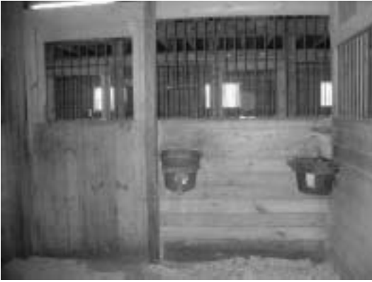
Figure 5.17. Stall with sliding door and separation of feed and water buckets. Water bucket is supplied by an overhead heated and insulated water line with individual valve to fill individual stall bucket.
