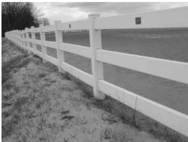
Figure 15.3. PVC rigid board fence is manufactured with the appearance of white board fence. PVC offers a low-maintenance fence but needs an electrified strand to withstand horse use.
