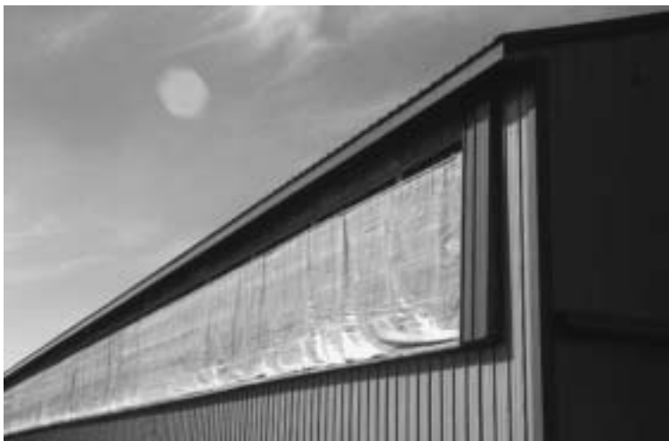
Figure 16.17. When closed, the translucent curtain sidewall material allows light entry but prevents wind entry. A continuous eave inlet opening is provided above the curtain.
