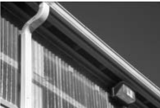
Figure 6.13. Riding arenas also need fresh air exchange year round, which is easily provided by eave inlet openings.
