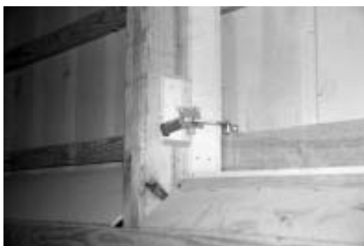
Figure 3.18. Durable latches provide tight closure of movable ventilation panels and large sliding doors.
