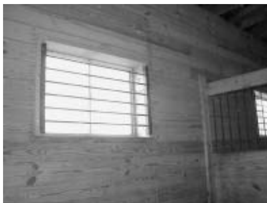
Figure 5.10. Protective bars on stall window.
