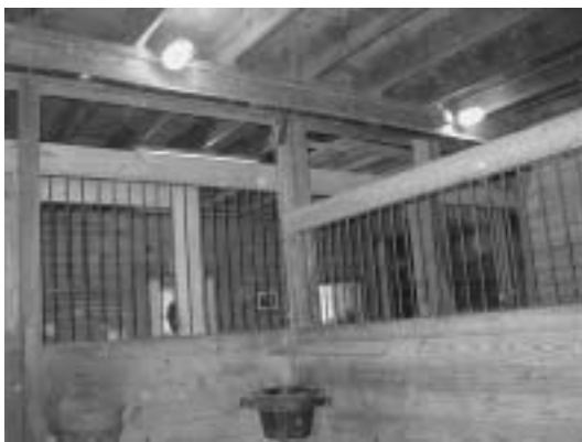
Figure 10.9. Water delivered in overhead pipeline with pull cord for dispensing water to individual buckets in each stall. Pull cord is accessible from work aisle. Water line is wrapped with electric heat tape covered with foam pipe insulation in freezing climate. Note electrical wiring protected in PVC conduit with sealed junction box. Incandescent stall lights are positioned at the front of each stall in a protective, sealed fixture. Aisle lights are fluorescent.
