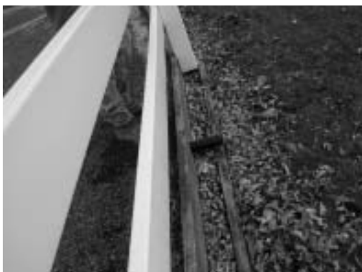
Figure 18.10. Boards may be used to help contain footing from leaving the arena surface. Gaps for water movement under the board will be needed. Shown here is a pipe moving water through the footing board. Lower board is supporting the base material above grade in a poorly drained location.
