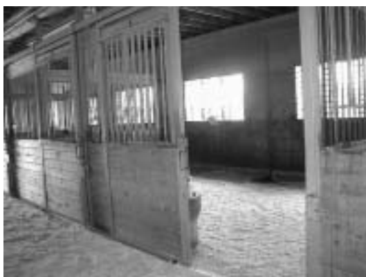
Figure 5.2. Interior partition removed to make one large stall from two regular-sized stalls. Large windows for plenty of natural light. Window glazing is removed for good air movement in warm weather.
