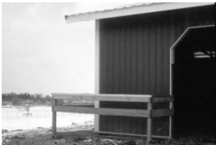
Figure 14.11. Fence horses away from contact with building exterior unless it is designed for horse contact. Metal-sided buildings need to have horses fenced away from the sheet metal that is easily dented by horse activity and will not withstand kicking abuse.
