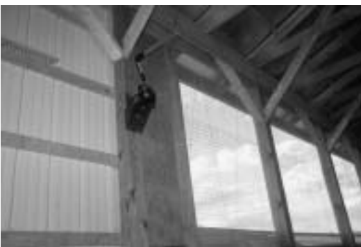
Figure 6.21. A hand-activated winch moves curtain up and down for less or more fresh air entry, respectively. Even with curtain closed, a 5-inch opening at eave admits fresh air during all weather. Curtain movement can be automated.
