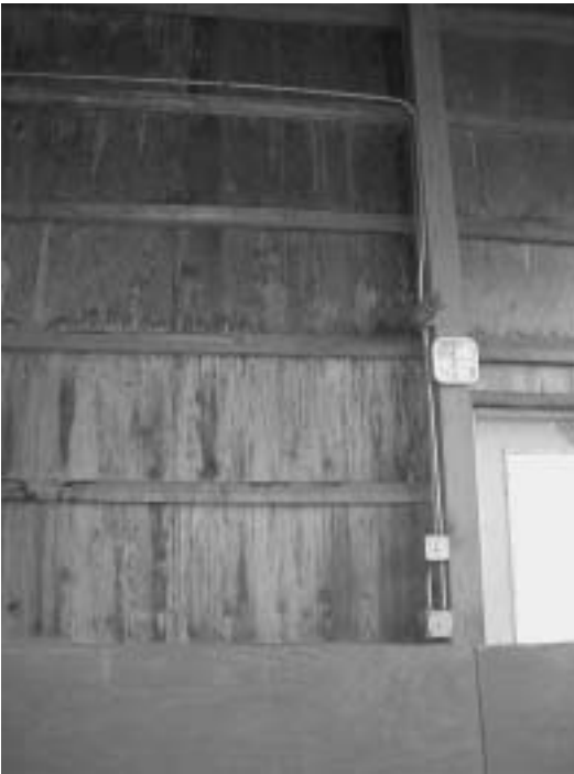
Figure 16.29. Use of moisture- and dust-resistant fixtures (not shown) and protected wiring in the indoor arena is necessary. Protection of all wiring at a height reachable by horses (up to 12 feet) is necessary, particularly in arenas where horses may be at liberty.
