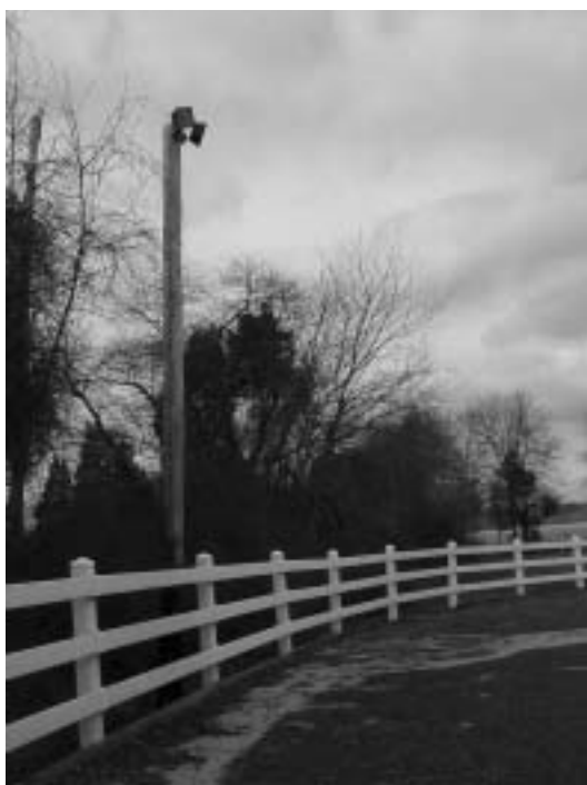
Figure 18.8. Mount HID lights on tall poles for providing at least a minimum amount of illumination without direct glare for night riding.
