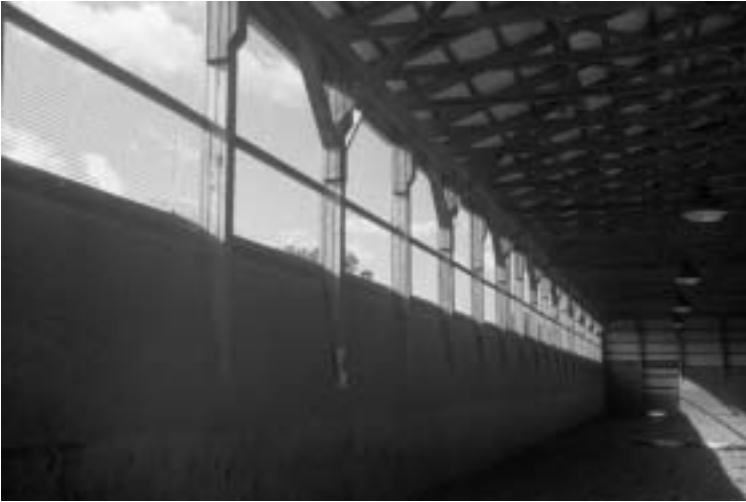
Figure 16.18. Indoor arena with curtain material on upper wall for abundant light and fresh air exchange. Bird mesh is provided to prevent bird entry at the curtain opening and as part of supporting the curtain when it is raised. Light entry and glare could be reduced through addition of shade cloth or other mesh material over the opening.
