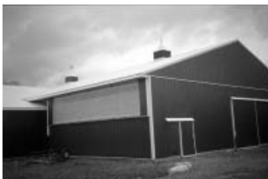
Figure 3.17. Curtain material along the top half of this riding arena's sidewalls is used for natural light entry and, when open, admits fresh air through the large openings.
