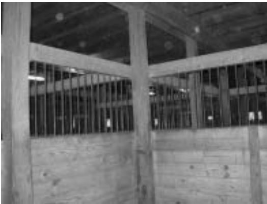
Figure 6.25. A double-aisle stable, which has four rows of stalls across the interior, has opened up the middle two rows of stalls with grillwork at the top of the stall walls and a relatively high ceiling. Fortunately, horses are turned out most of the time. Allowance for air distribution throughout the middle portion of this stable design is particularly important because these stalls do not have direct access to fresh air as the outer stalls along the sidewalls.
