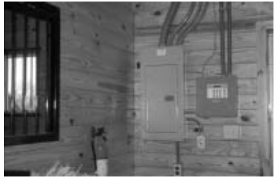
Figure 10.4. Electrical service panel located in unheated storage area on endwall of stable with easy access from outside door. Note handy fire extinguisher.
