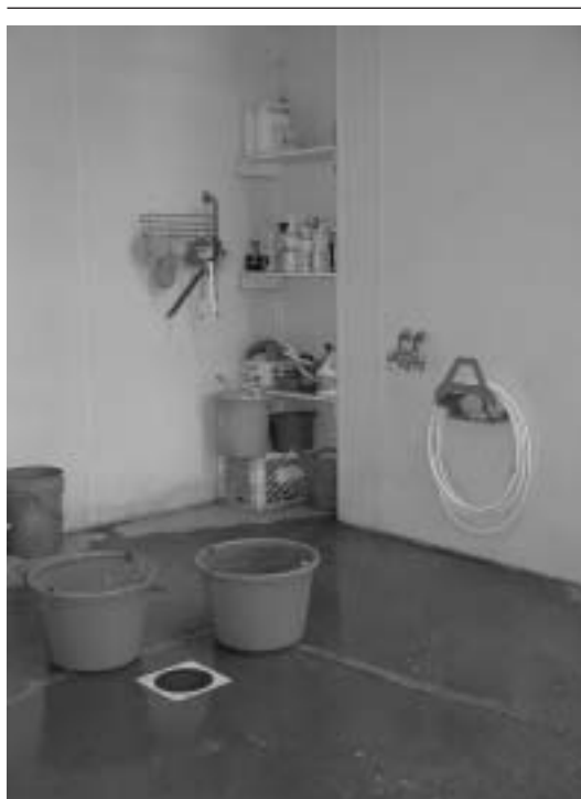
Figure 13.17. Wash stall with recessed shelving in back corner. Wall material is FRP, which is strong and waterproof.
