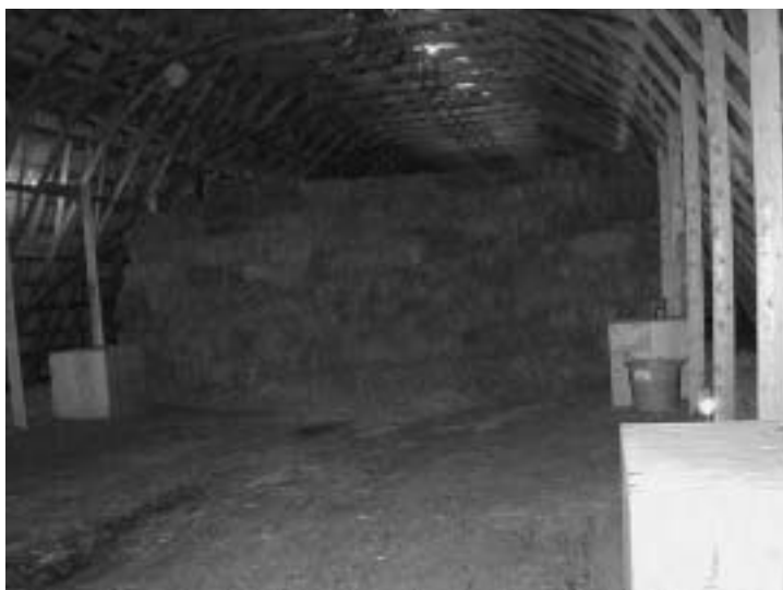
Figure 13.5. Haymow long-term storage that provides air circulation around and over the stacked hay. Plywood boxes cover hay drops to stalls below.
