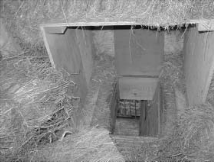
Figure 13.7. Interior of plywood box covering hay drop hole for two stalls below. Hinged lid, toward back of box, can be closed to protect hole further. Hinged baffle is directed to right to send hay delivery to stall on left.
