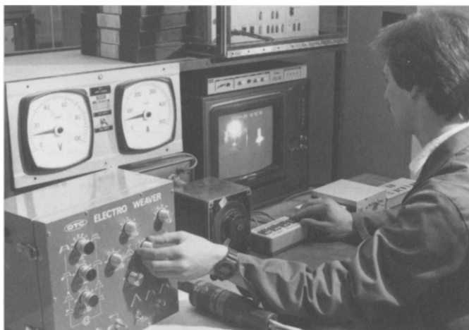
38 Remote controlled welder in use at The Welding Institute.
