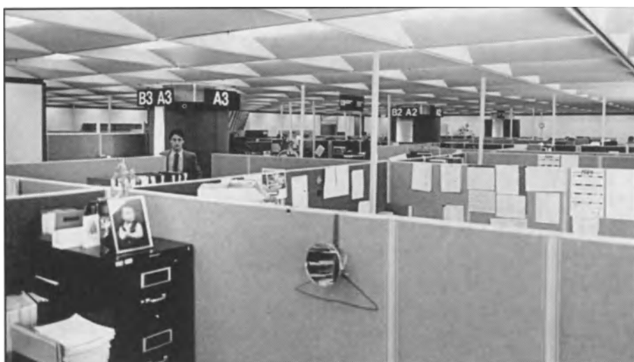
Figure 7.2. Typical coffered ceiling configuration, with two-bulb fixtures behind acrylic lenses.
