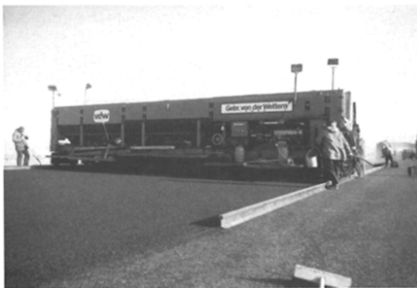
Fig. 8.6 11.5 m gussasphalt screed bar train
