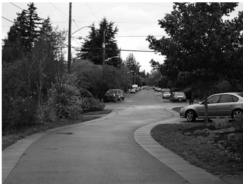
Figure 5.3.1 The Street Edge Alternative (SEA Street) in Seattle, Washington is a natural drainage system (NDS) designed to direct street run-off from a narrowed street pavement to planted infiltration swales. Note the adjacent street in the background showing the pre-SEA Street condition with wider road pavement and conventional stormdrains. Photo: Jack Ahern
