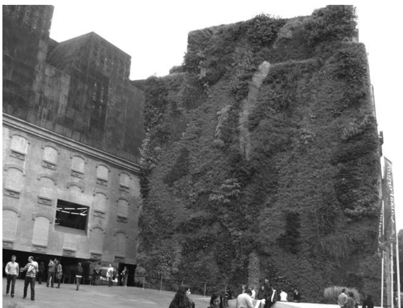
Figure 5.6.2 The 'green wall' at the CaixaForum culture forum on the Paseo del Prado in Madrid, which covers some 460 m 2 and supports 15,000 plants from 250 different species. Copyright: John Box (author)
