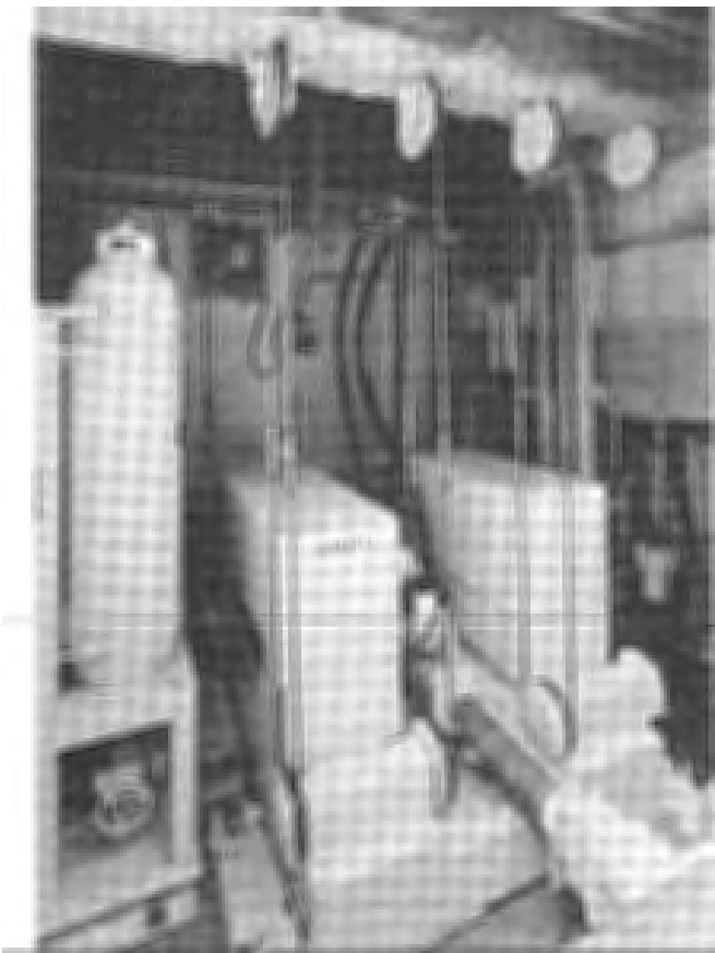
Figure 5.27 View of active mass driver in Kyobashi Seiwa building (courtesy of Kajima Corporation, Tokyo, Japan)
